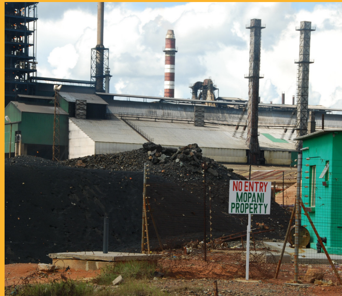
Mufilira mine consists of an underground mine, a concentrator, a smelter and a refinery.
