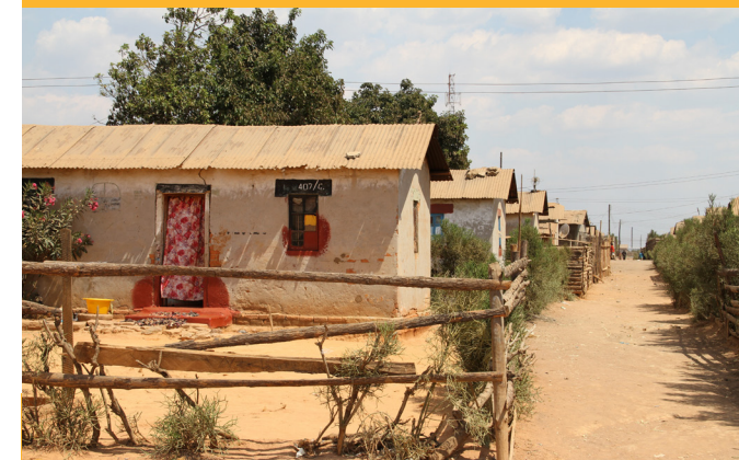
In Kankoyo, the roofs and paints on houses are corroded by the acidity
